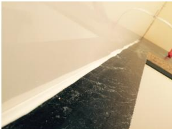
New splashback is to be laminated on all edges to stop water penetrating splashback. Excess sealant is removed on completion.
